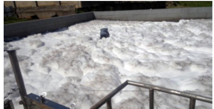
Waste water foaming before Chemical Leasing
